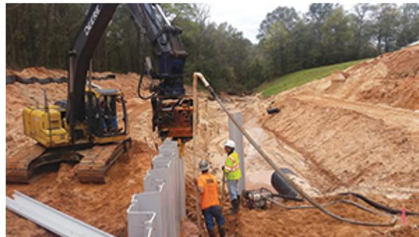
Sheet piling was used to create a stilling basin to slow water velocity.
